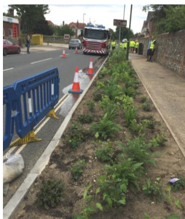
One of the two Littlehampton rain gardens on Maltravers Road.
